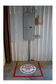
There shall be no knock outs in the box that are open. Every breaker should be clearly marked.
